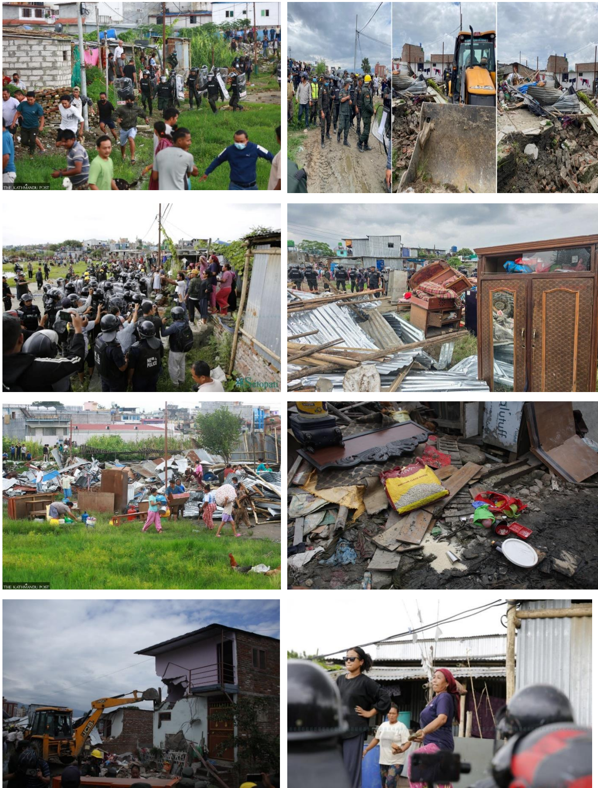
Figure 5. Bulldozer demolition after clash and eviction in Manohara Squatters Settlement
